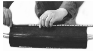
Installing shrinkable sleeve, slide on channel
