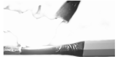
Tightly wrap one half-lapped over cardboard liner with adhesive tape
