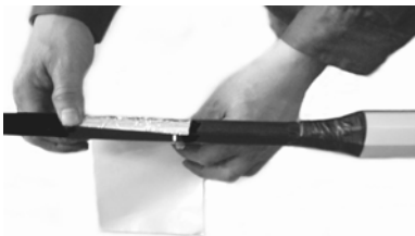
Wrapping aluminum foil strip over mark 10mm
