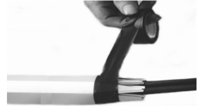
Tightly wrap one half-lapped over cardboard liner with adhesive tape
