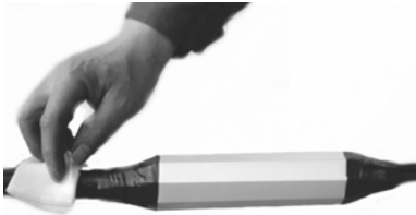
Applying desiccant and continuity wire, tightly wrapping closure with PE pack-bag
