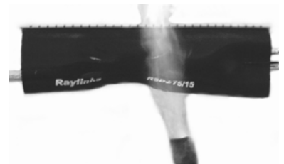
Continue heating evenly around sleeve from center to end until entire sleeve is recovered
