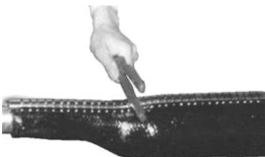
Tap channel down to conform to cable
