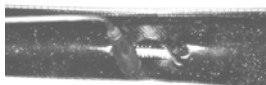
Continue heating evenly around sleeve from center to end until entire sleeve is recovered
