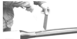
Abrade the cable sheath circumferentially On the cleaned area with the abrasive strip
