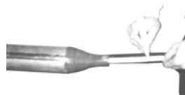
Place a mark on the cable just outside the edge of the sleeve
