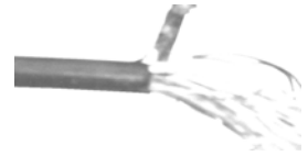
Attach shield continuity wire to cable sheath with clip.
