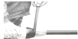
Tightly wrap one half-lapped over canister with adhesive tape
