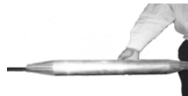
Center the metal canister over splice
