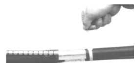
Strain cables with tie wrap
