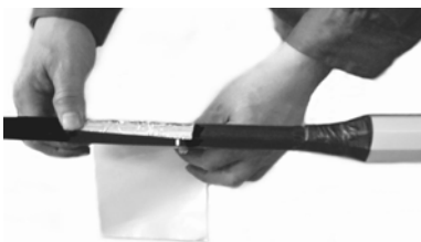
Wrapping aluminum foil strip over mark 10mm
