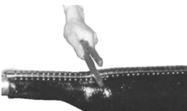
Tap channel down to conform to cable
