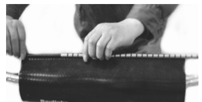
Installing shrinkable sleeve, slide on channel
