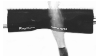
Continue heating evenly around sleeve from center to end until entire sleeve is recovered
