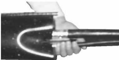
Wrapping aluminum foil strip over mark 10mm
