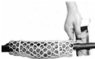
Wraps around the cable edge with Mastic strip
