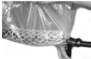
Wrap around joint with transparence film, tight wrap the edge on mastic with PVC type.
