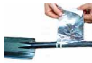
Make the aluminum foil conform to cable
