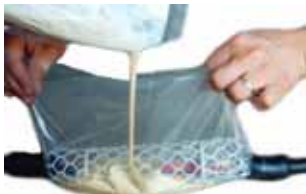
Fill sealing resin to top of mesh
