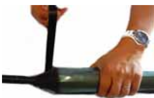
Tightly wrap one half-lapped over canister with adhesive tape
