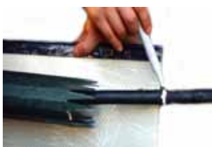
Place a mark on the cable just outside of the edge sleeve
