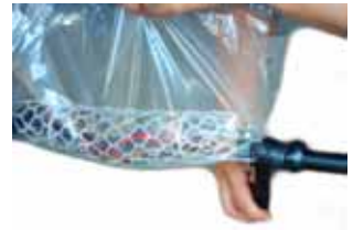
Wraparound joint with PE package, tight wrap the edge of it.
