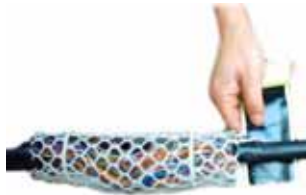
Tight wraps the edge of mesh with adhesive tape
