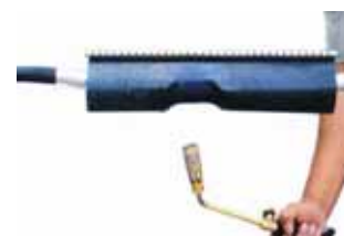
Continue heating evenly around sleeve from center to end until entire sleeve is recovered
