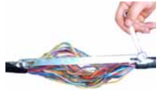
Install the shield bracket
