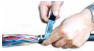
Tight wraps the edge of cable with adhesive tape.
