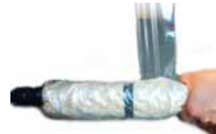
Tight wraps with PE package
